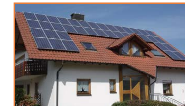
Off-grid home solar system
