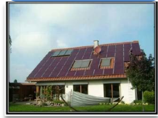
Residential Rooftop PV system
