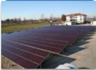
Ground mounted PV system
