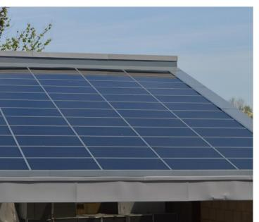
Polysolar's black opaque thin-film PS-CT series is a high efficiency panel with side or back connectors
