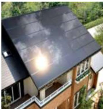
**Polysolar's PS-M-NX opaque and transparent panels incorporate micromorph technology to achieve high efficiencies and aesthetic design.**
