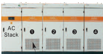
DC stack (250KWx4=1,000KW)
