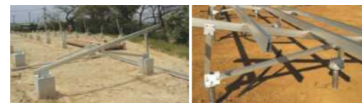
Concrete foundation
