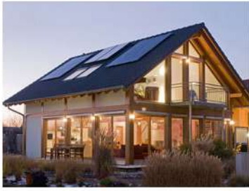
Home photovoltaic system
