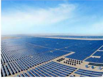
Photovoltaic power station
