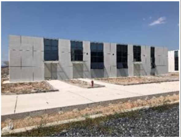
PCS, DCP, ACP, Control Box Assembling Line
