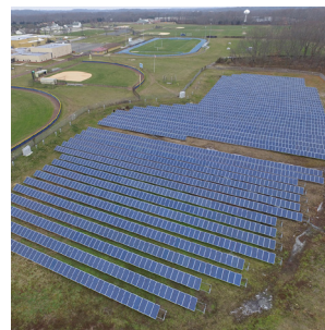
2 MW - Plumsted School New Jersey
