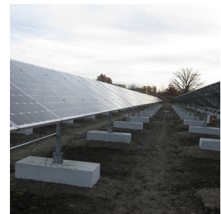
1.2 MW - Marysville Michigan
