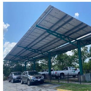
1 MW - Washington District of Columbia
