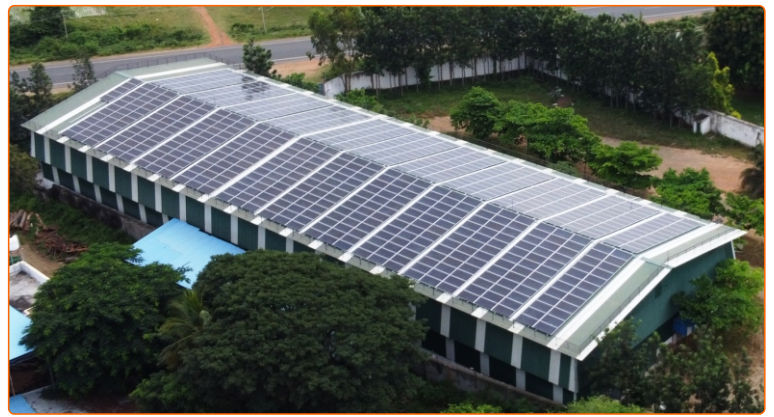
Rooftop Solar System
