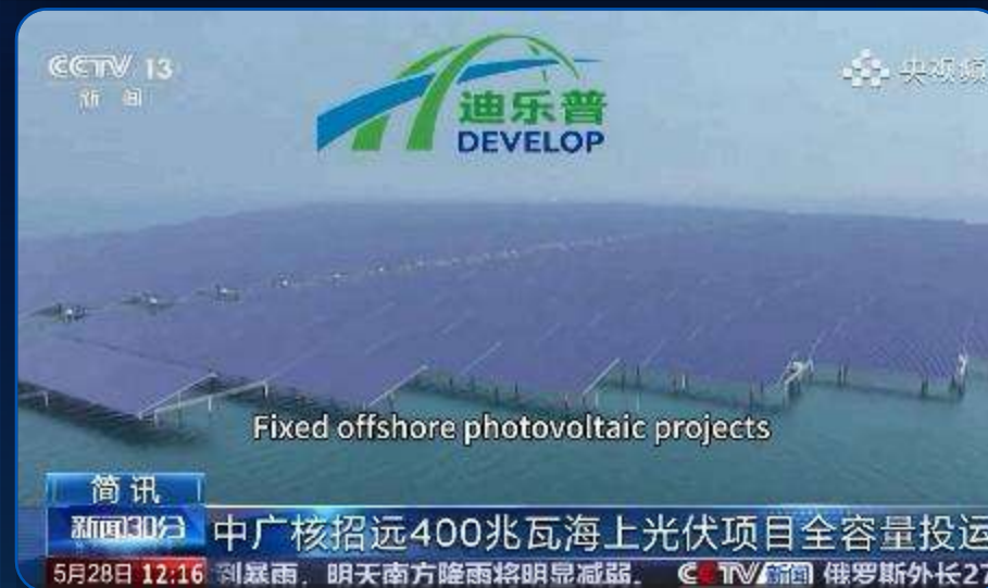
Project Site: CGN Zhaoyuan Offshore PV Farm
