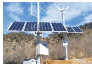
Base station/cell tower
