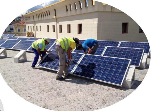
SOLARBLOC® removes the process of metal structure mounting and weighting or anchoring.
