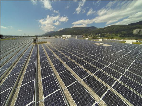
**Aerodynamic south oriented mounting system for flat roofs**
