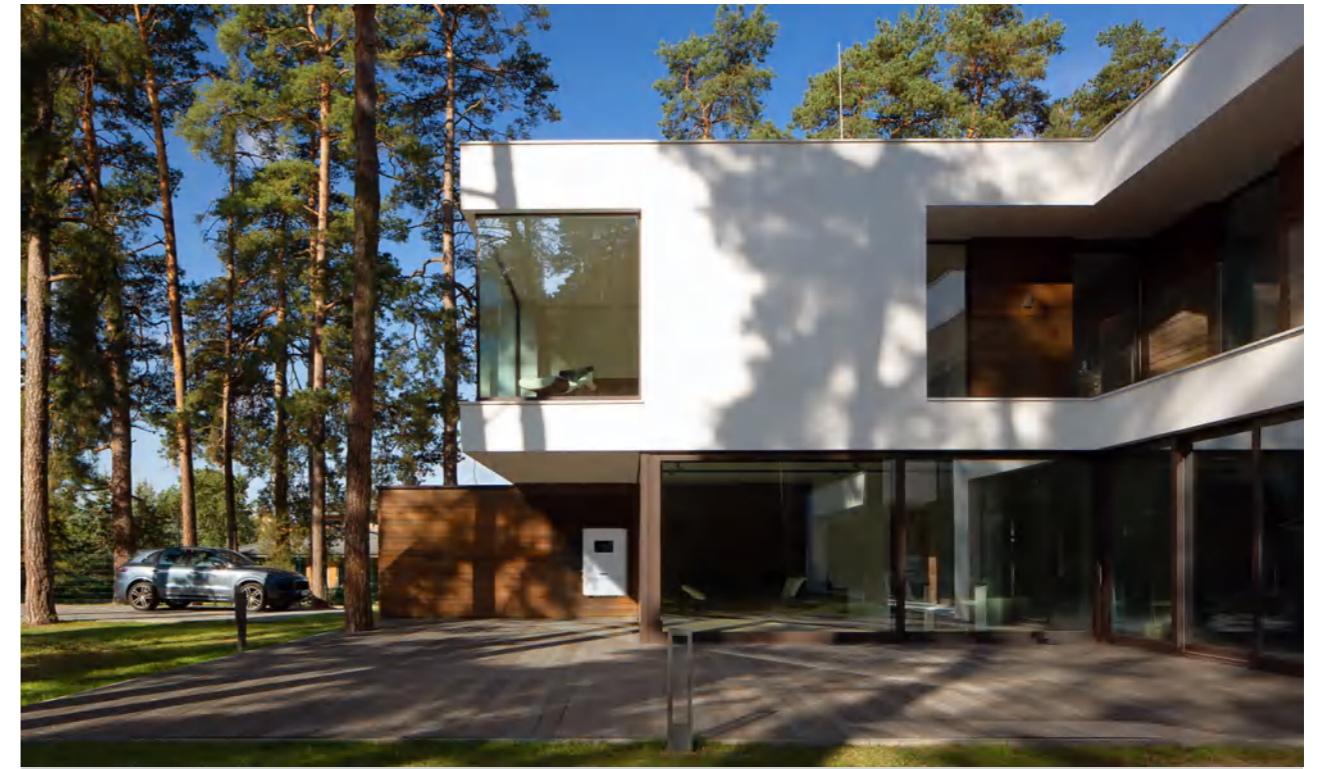
Residential Project in the United State 10kW
