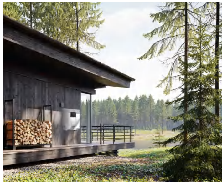
Residential Project in Estonia 8kW
