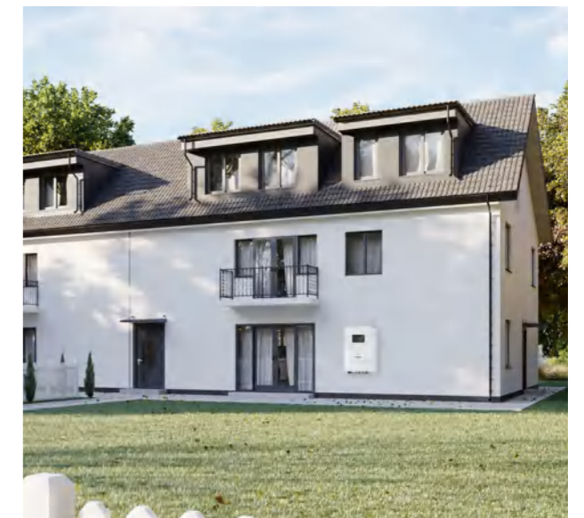
Residential Project in the United State 6kW
