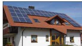
Off-grid home solar system
