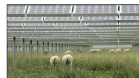
Farm solar generation system
