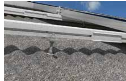
Installation on corrugated roof
