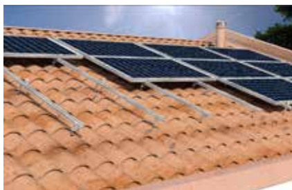
Installation on tiles roof
