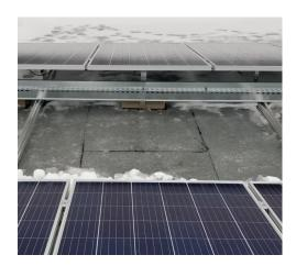
Rails provide effective cable management opportunity and design allows easy access to panel junction box and PV cables
