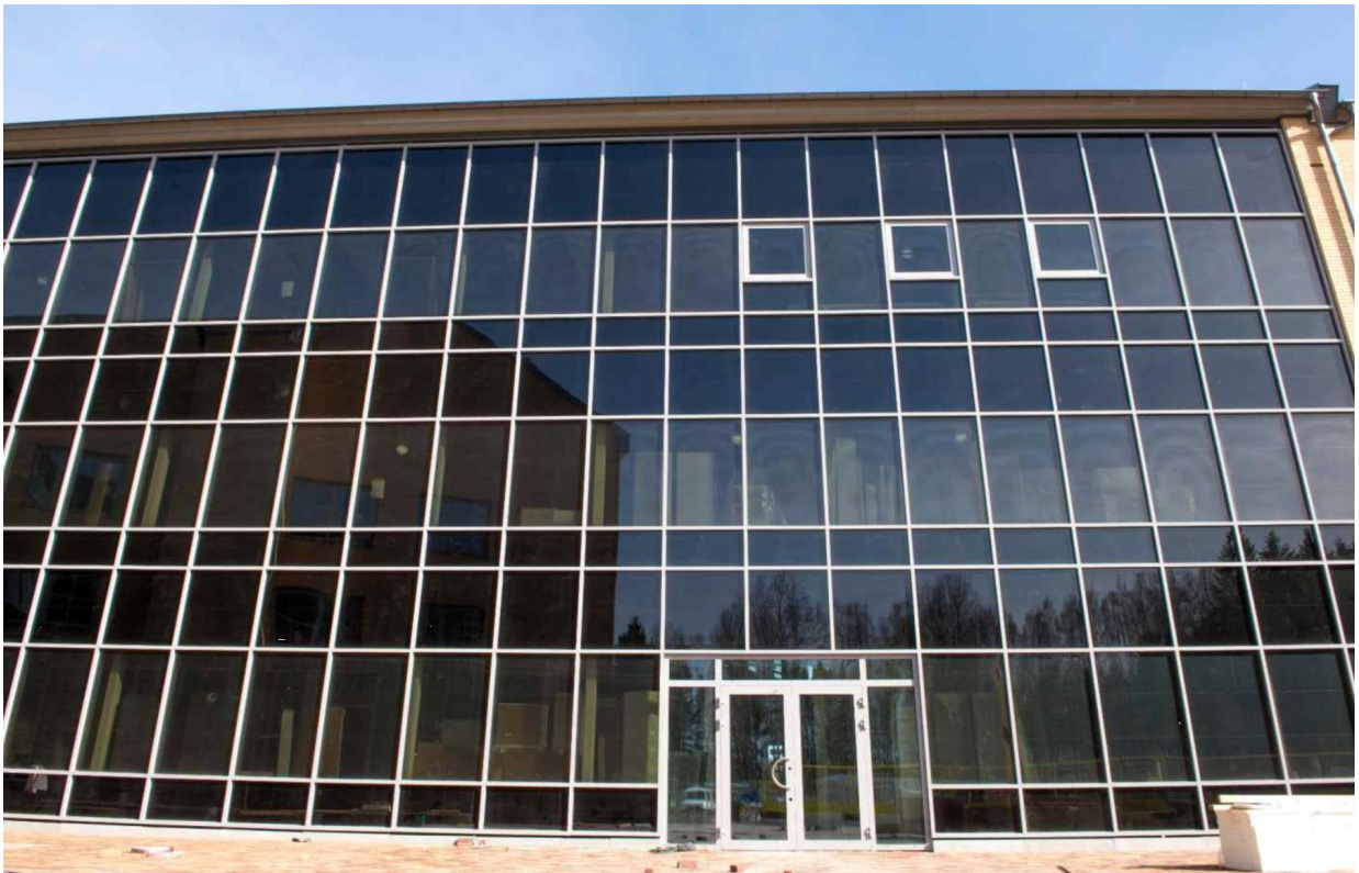
BIPV Glass Curtain Wall, UK
