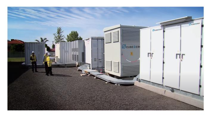
Cubenergy FlexCombo-M30 is designed for community microgrid and min Commercial& Industrial application. The solution is an organic combination of renewables and BESS, which unlocks lower-cost energy supply while increasing the use of renewables in rural districts, remote areas and islands. The FlexCombo solution offers reliable microgrid and energy storage tailored to suit the ecological sensitivities of remote site economies.
